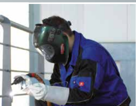
2. Steel / stainless welding in DC
